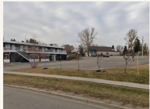
Allendale Road frontage.
